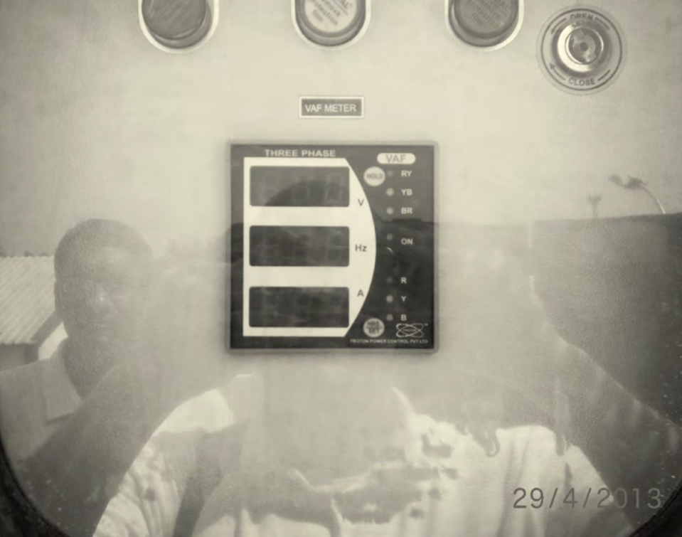
UNSTABLE GRID The PV inverters' AC collector shows what is currently happening in the utility grid.
