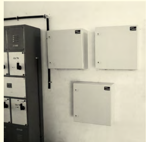
INTERFACE The SMA Fuel Save Controller integrates photovoltaics into the diesel power grid. This enables Alpine Knits to save 50,000 liters of fuel per year.
