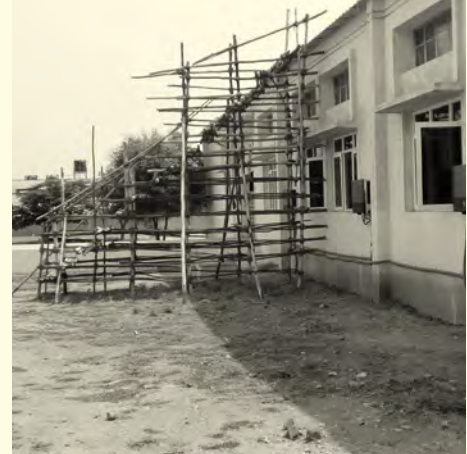
SOLAR PLANT CONSTRUCTION - INDIAN STYLE Via a bamboo staircase, modules and inverters for the PV system are transported onto the roof of the factory.
